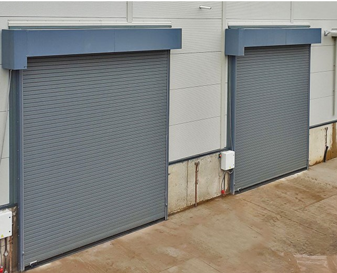
Insulated roller shutters, externally mounted in powder coat finish with matching roller and motor hoods
