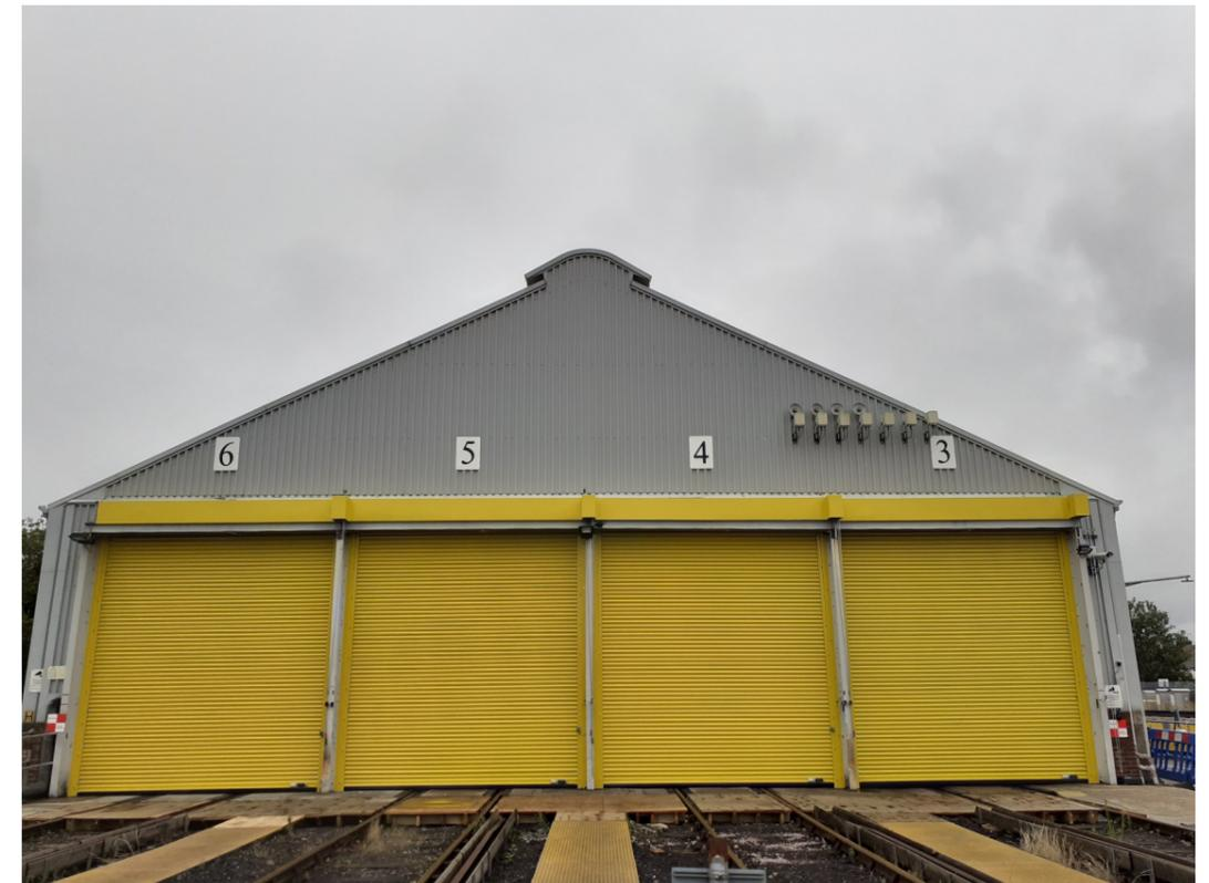
Roller shutters to railway shed in powder coat finish and non insulated lath profile..
