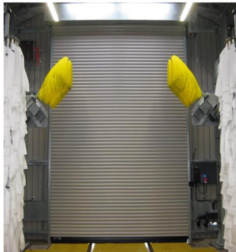
Electric roller shutters are versatile doors and can be applied in various harsh environments with only slight modifications. Shown above is an electric roller shutter fitted internally to a train wash station. Enclosures, specially protected electronics allow this door to be frequently exposed to the water and solvents used in cleaning.
